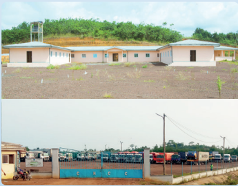
CNSC Dibamba Trucker Accomodation Centre Littoral Region
