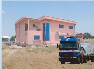
CNSC Kousseri Trucker Accomodation Centre Far-North Region
